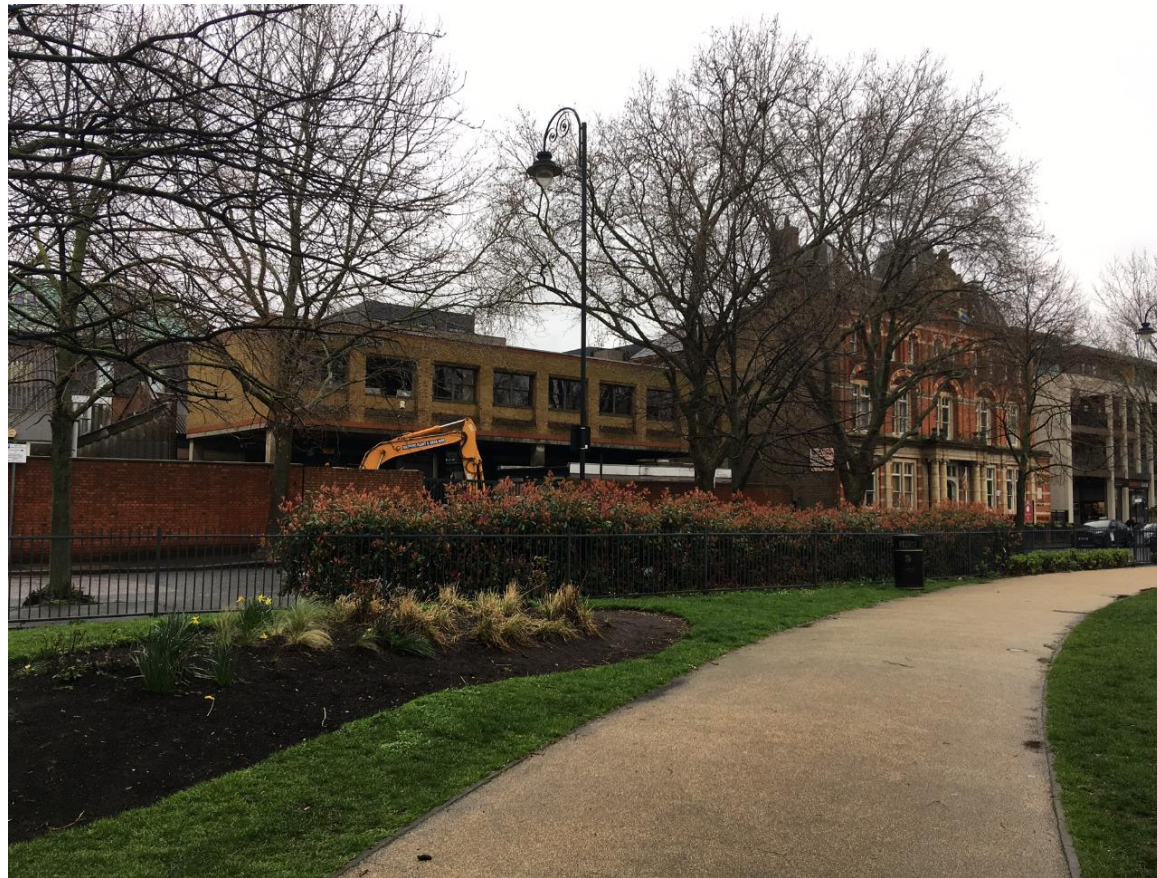
Looking east towards site
