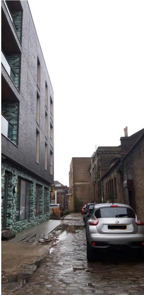
Looking east towards site from Grange Yard
